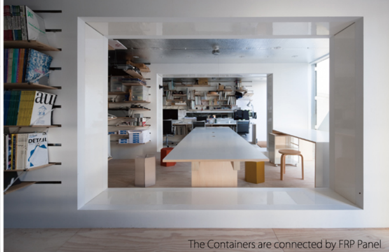
The Containers are connected by FRP Panel
