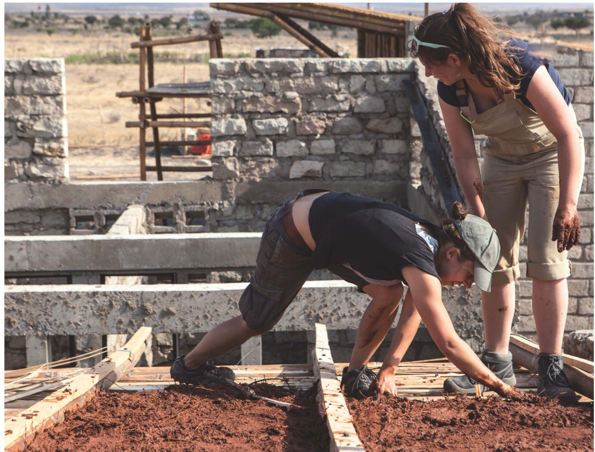
dormitory roof construction with clay cover, photo © M.Kestel
