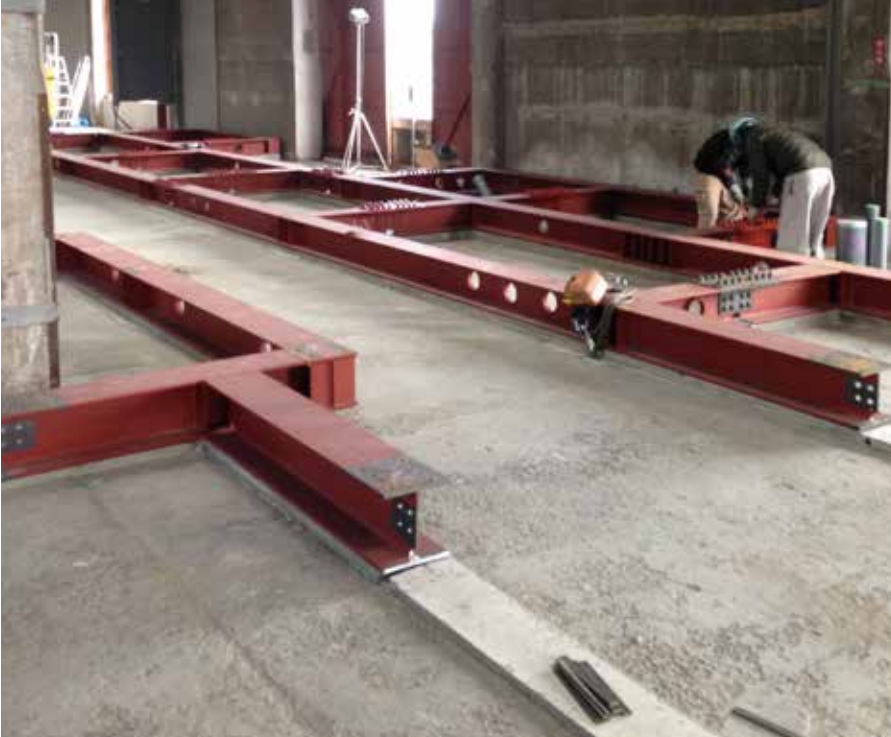
Step1:put steel beams on the mortar. This works instead of the RC base.
