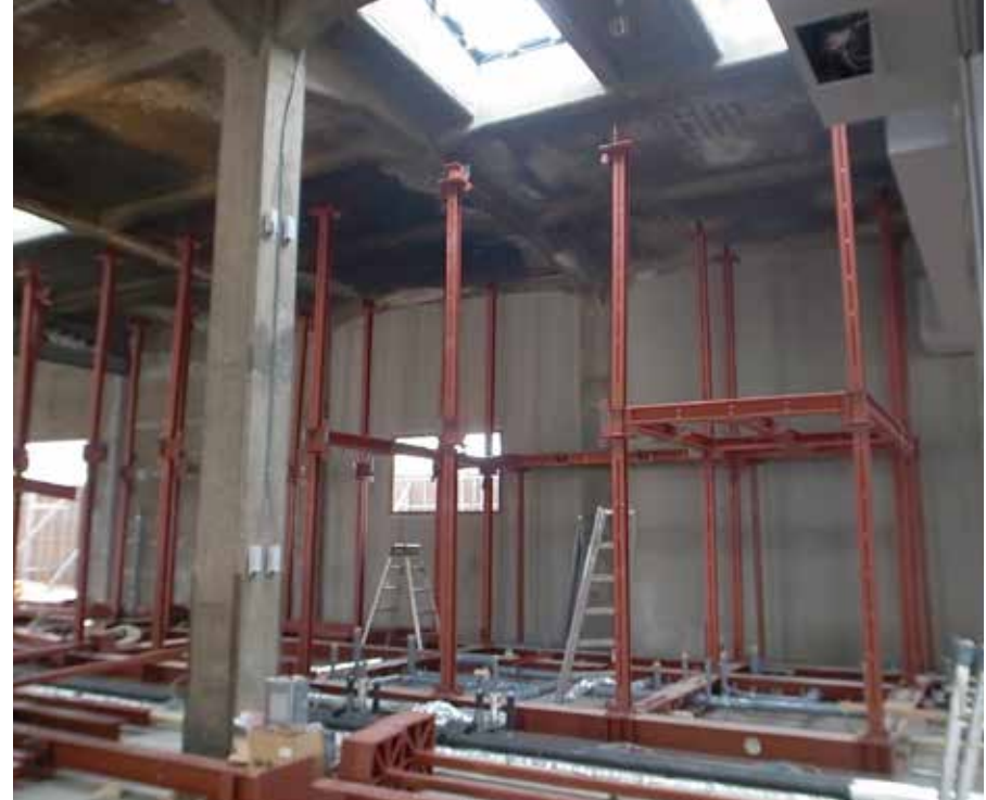
Step3:Fix the structures with the beams. We can put beams close to the ceiling.
