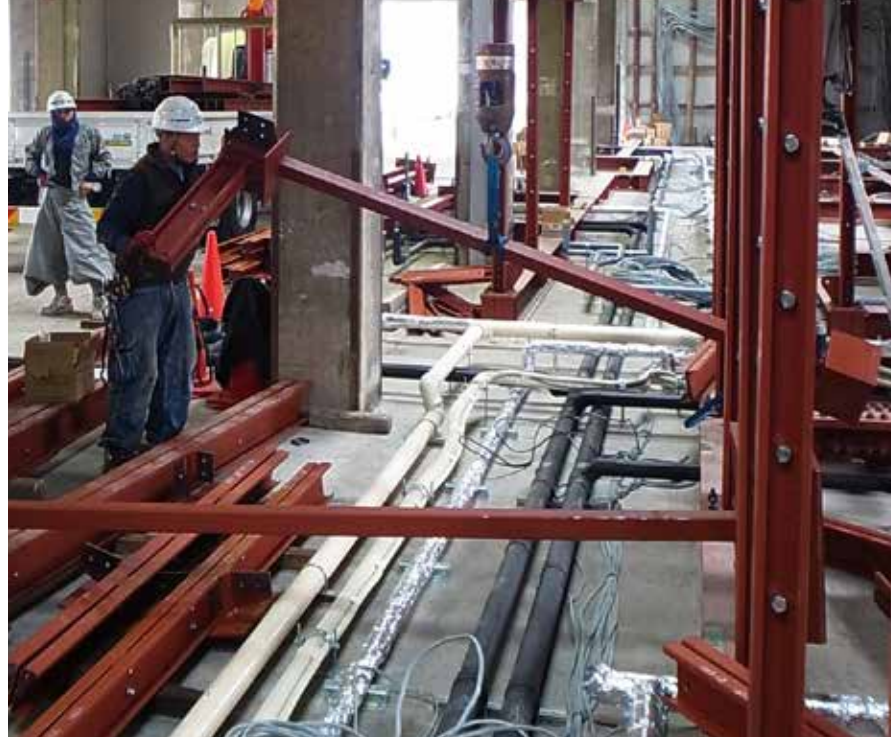
Step2:Put the LGS structures on the beam with machine and humuan.
